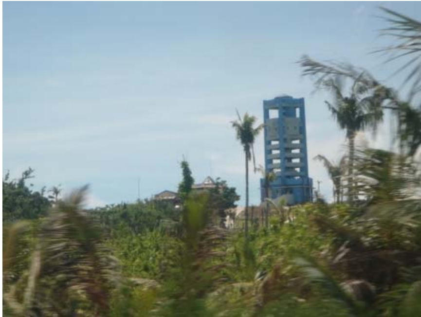
Guiuan radar (antenna was blown out)
