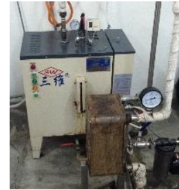
Existing Electric Boiler
