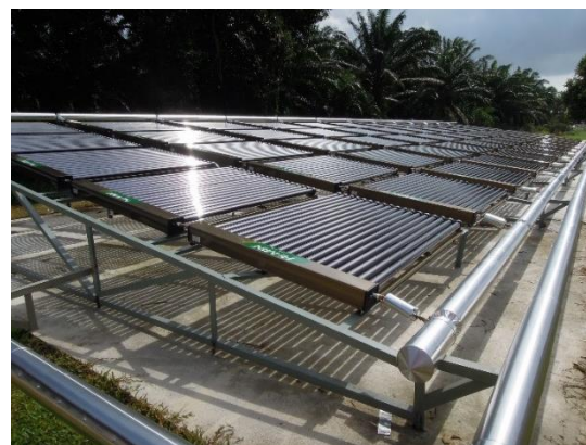
Solar Thermal Collectors
