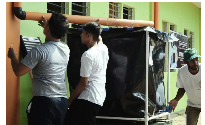
Installation and connection to downspout of a building.
